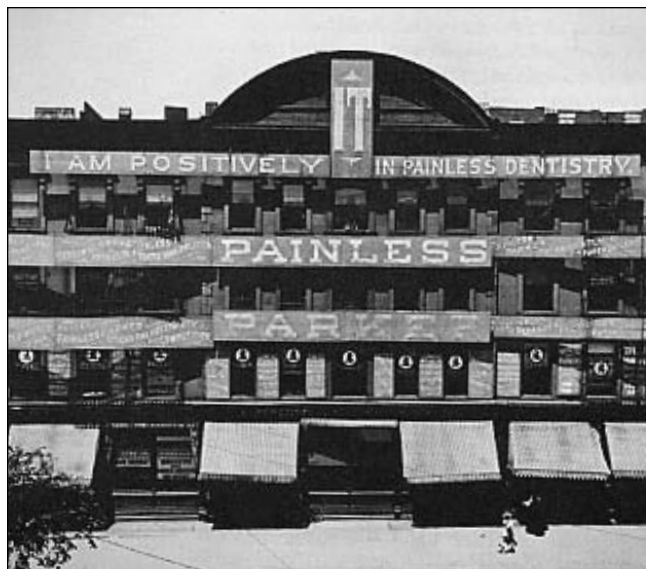
Fig. 7—Parker's Flatbush Avenue office in about 1900.
